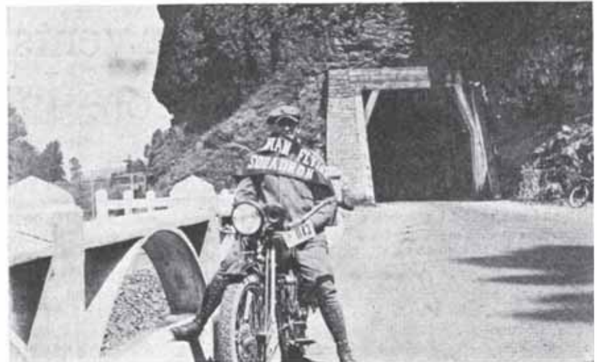
The tunnel pierces a wall of solid rock
